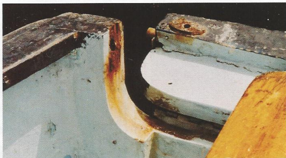
Despite the rusty appearance these security bolts still work after six years
