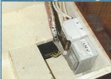
20: Completing the cabling
